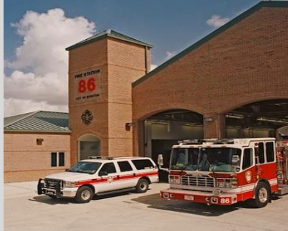
Houston Fire Department Fire Station #86, Houston, TX
